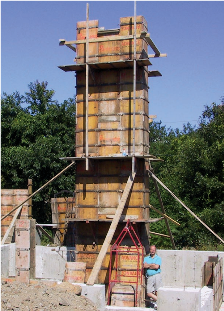
Built at the same time as the house's foundation, a massive 23-foot-tall pier of reinforced concrete provides a stable base for the telescope even when there is considerable activity in the adjacent rooms.
