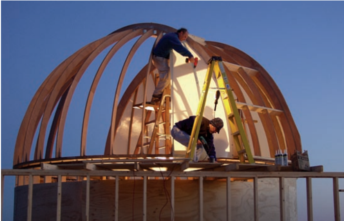
Left: After six months of making parts for the dome, the author enlisted the help of a dozen members from the Amateur Telescope Makers of Boston for a “very long weekend” spent assembling the dome atop the observatory walls. Right: The telescope’s pinpoint star images are apparent in this image of the globular star cluster Messier 13 in Hercules.
